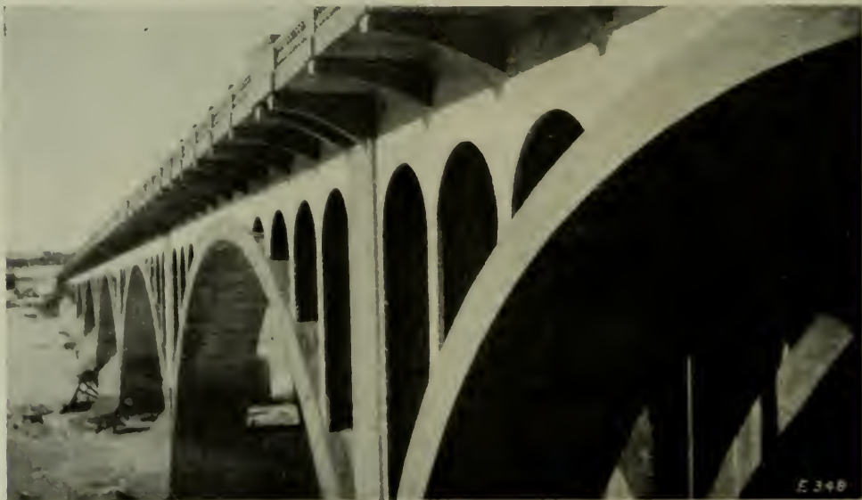
REINFORCED CONCRETE BRIDGE AT SASKATOON.
